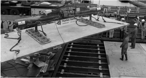
Figure 3. Placing of heavy-reinforced UHPC panel in motorway 44 near Sassenheim. (the Netherlands).
