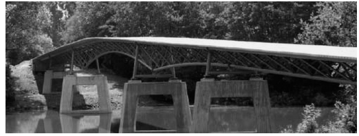
Figure 5. Gärtnerplatzbridge composite steel-UHPC bridge at Kassel (Germany).
