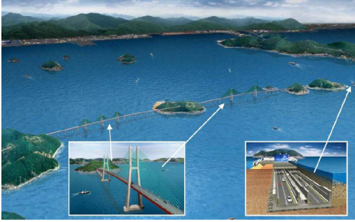
Figure 3. Busan-Geoje Fixed link with bridges and immersed tunnel designed for 100 years' service life using the full probabilistic service life approach following the fib Bulletin 34.
