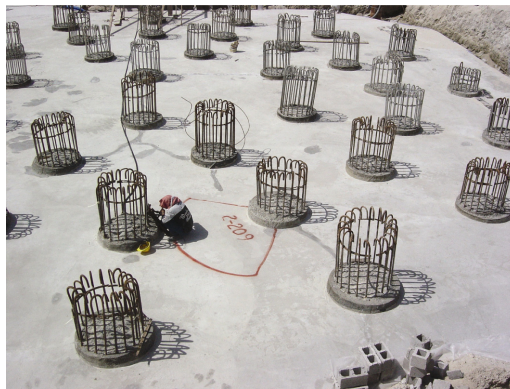
Figure 6. Qatar Nation Library, piles and foundation elements. Reassessment of service life.
