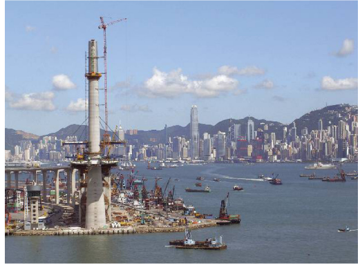
Figure 8. Stonecutter Bridge, Hong Kong. Design: COWI A/S in joint venture with Arup.
