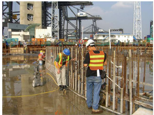
Figure 9. The outer layer of reinforcement of the Stonecutter Bridge is stainless steel. The remaining is ordinary black steel.
