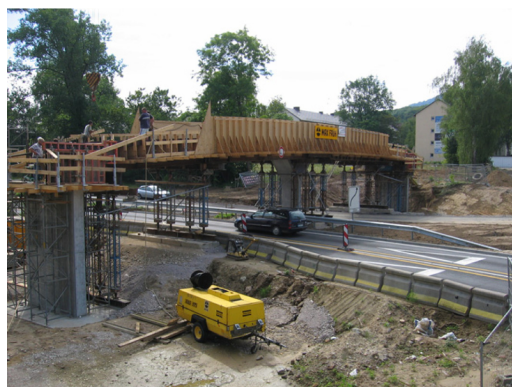
Figure 9. On-site construction of the concrete deck.
