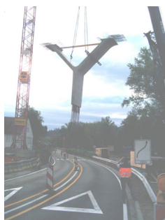
Figure 8. Column is moved by a crane to its place.
