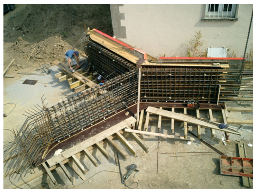
Figure 7. Formwork and reinforcement for the Y-shaped column laying on side.
