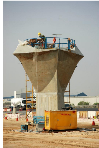
3-span unit central pier cap
