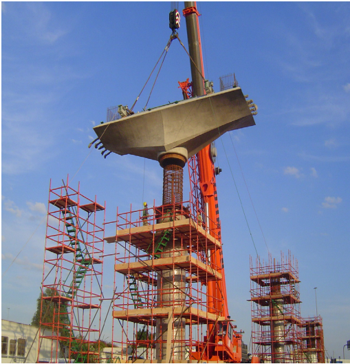
Lifting of a pier cap shell
