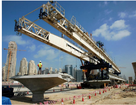
Erection of a simple span
