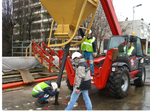
Photo 4. Pouring by pouring channel.
