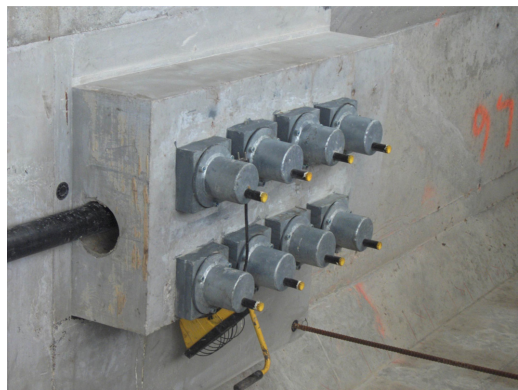
Photo 6. Anchor block anchorage by bars.
