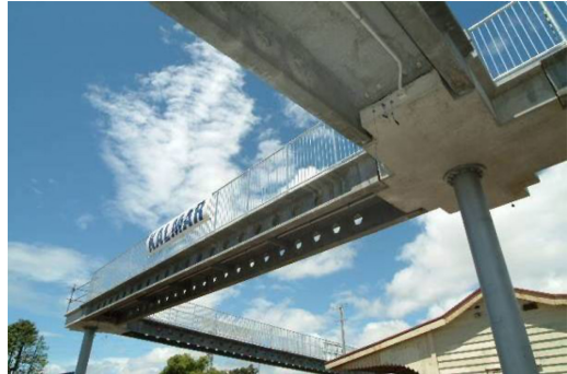
Figure 16. Penrose Footbridge during construction.
