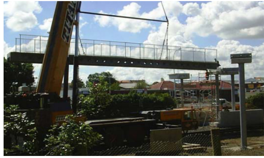
Figure 15. Ductal® span with railing attached being lifted.
