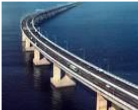
Rio-Niteroi Bridge (RJ)
